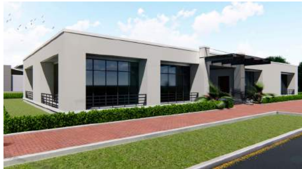
Startup Research Building
